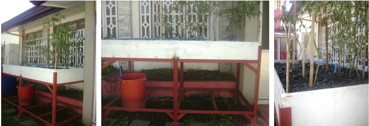
New metal frame and grow bed for the aquaponics system – there is room underneath for the new fish tank that we will make in the future.
